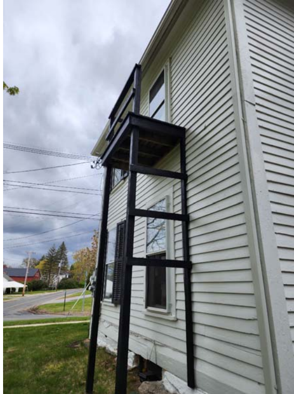
Photograph #9 (Town Hall Annex) – Exterior Fire Escape
