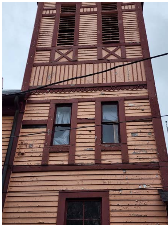
Photograph #20 (Town Hall) – Exterior Wood Siding & Trim
