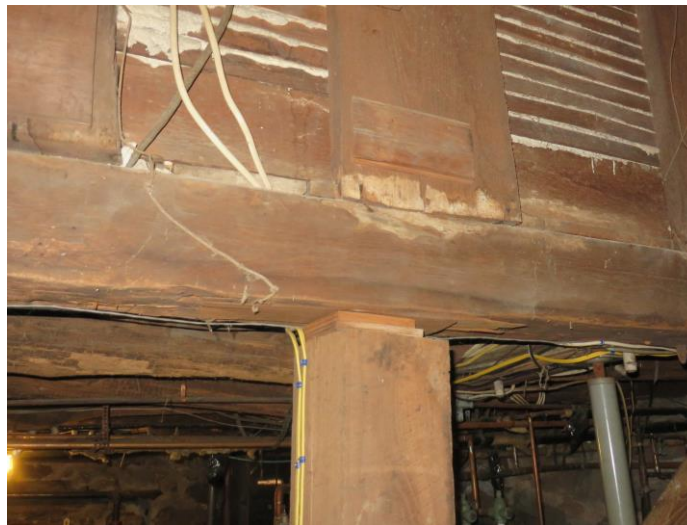
Photograph #20 – First Floor Beam-Column Connection
