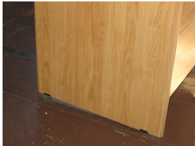
Photograph #11 – “Treasurer” Sloped Floor
