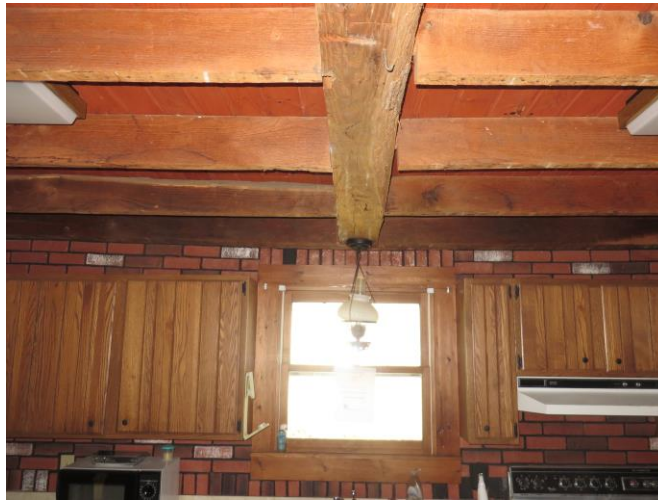
Photograph #7 – “Kitchen” Ceiling/Attic Framing
