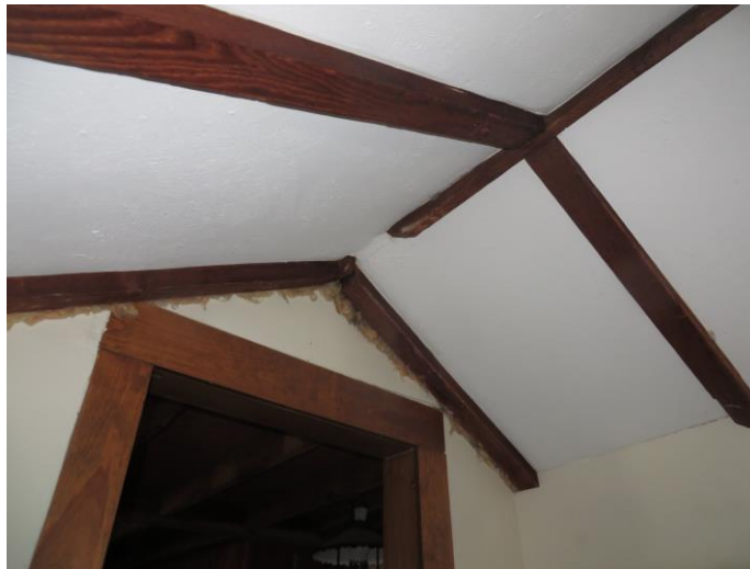
Photograph #5 – “Storage” Ridge Member
