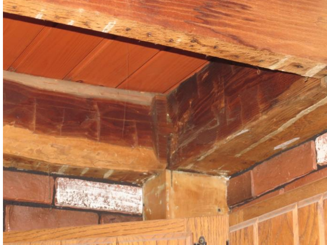
Photograph #8 – “Kitchen” Beam-Beam Connection
