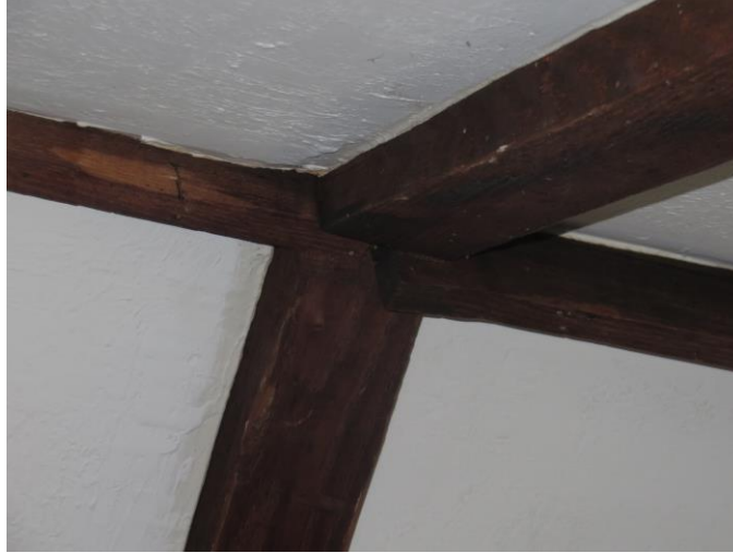
Photograph #4 – “Storage” Ridge Member
