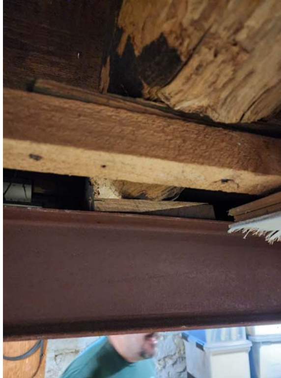
Photograph #7 (Town Hall Annex) – Wood Blocking Above Shoring
