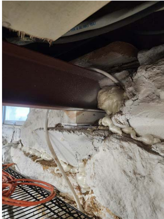
Photograph #5 (Town Hall Annex) – Shoring Beam Bearing
