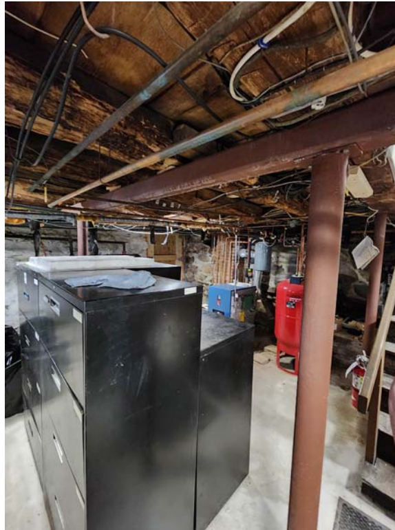
Photograph #1 (Town Hall Annex) – First Floor Shoring
