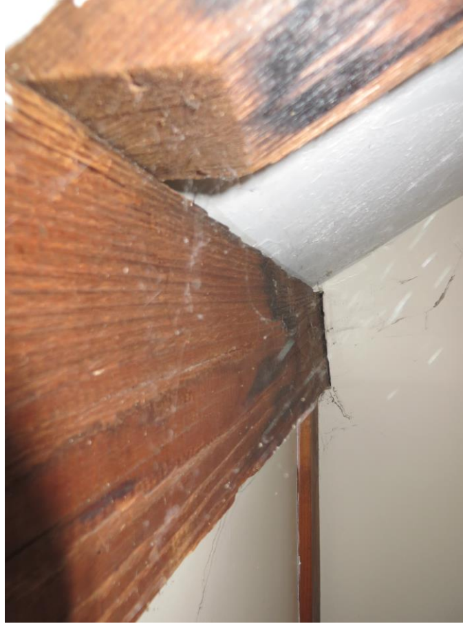
Photograph #6 – “Storage” Perimeter Roof Beam
