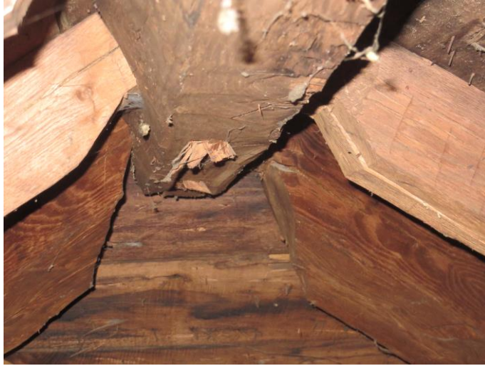
Photograph #1 – Existing Roof Framing (Original Building)
