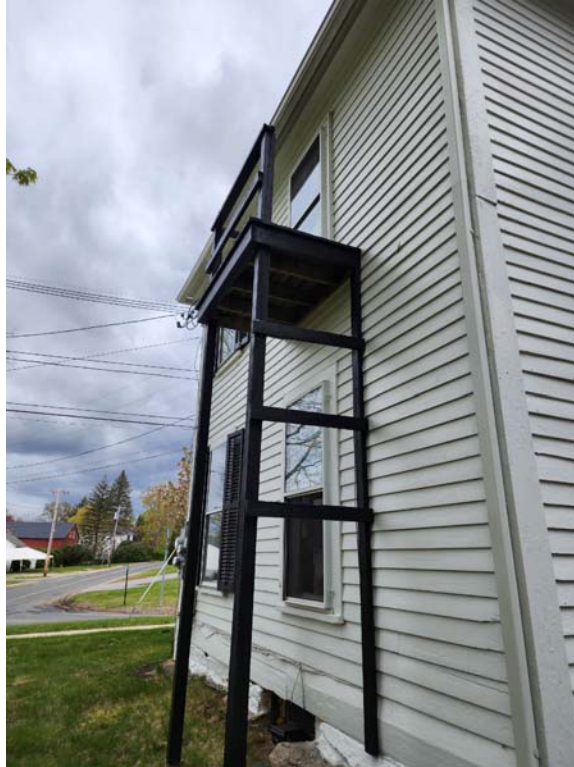
Photograph #9 (Town Hall Annex) – Exterior Fire Escape
