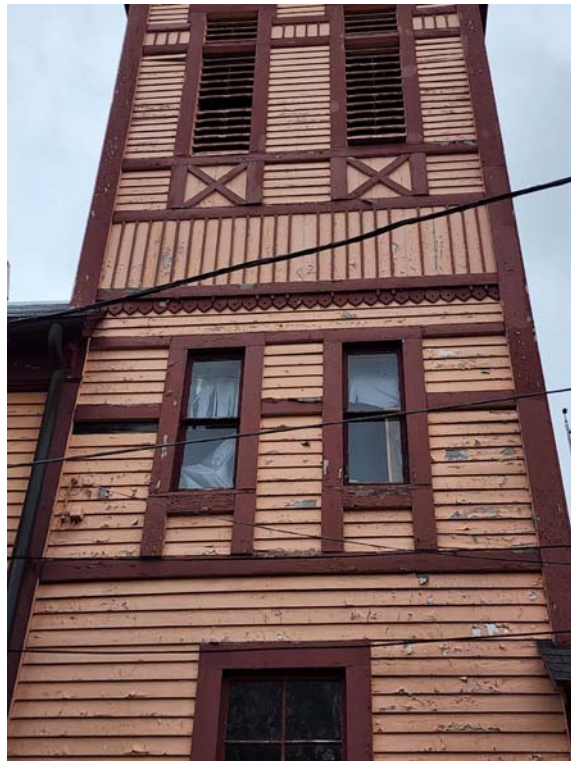
Photograph #20 (Town Hall) – Exterior Wood Siding & Trim
