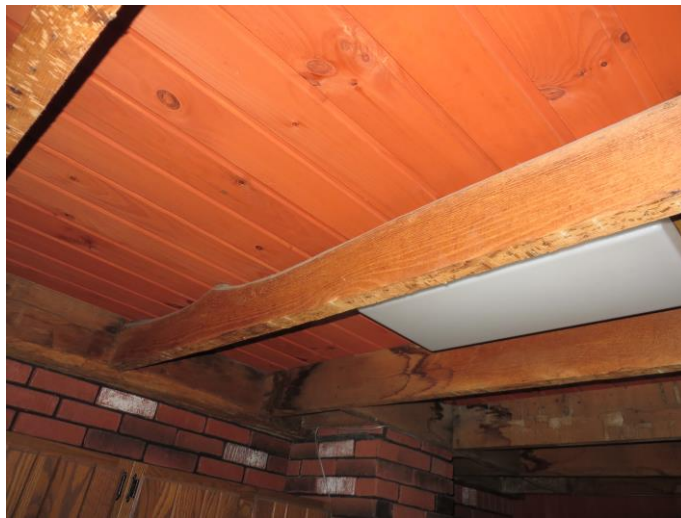
Photograph #9 – “Kitchen” Ceiling/Attic Joist
