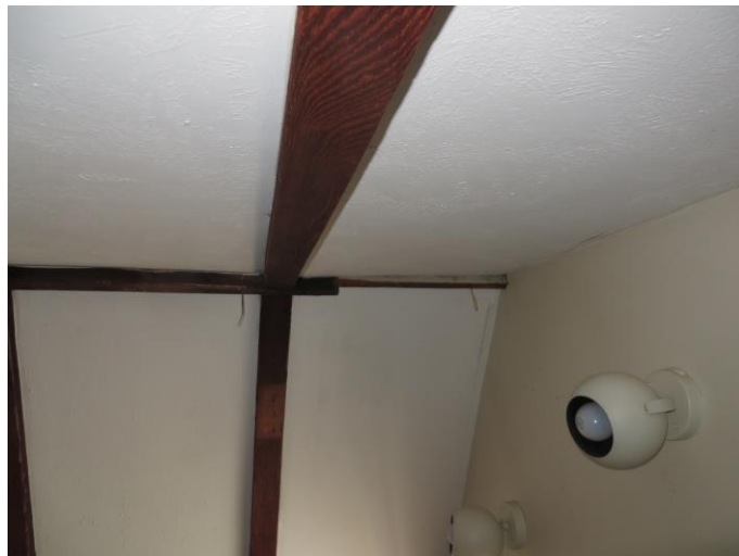
Photograph #3 – “Storage” Ridge Member
