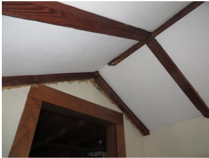
Photograph #5 – “Storage” Ridge Member
