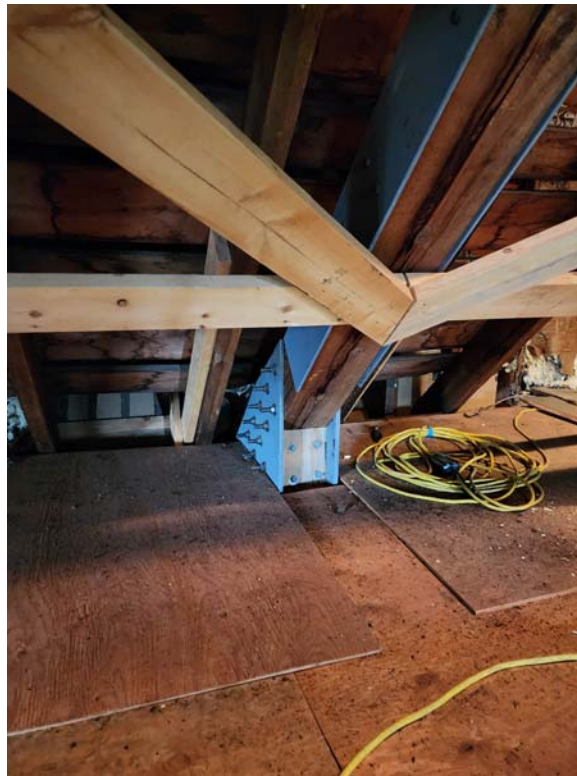
Photograph #24 (Town Hall) – Reinforced Roof Truss Member
