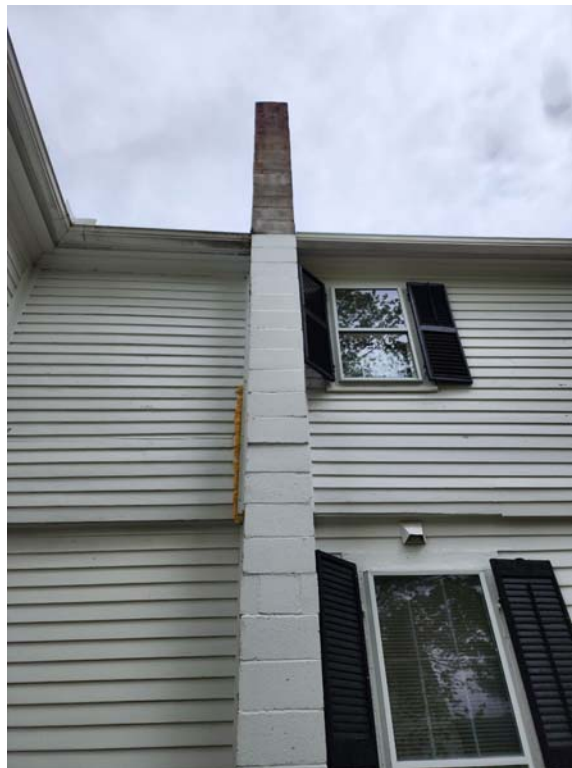
Photograph #8 (Town Hall Annex) – Chimney
