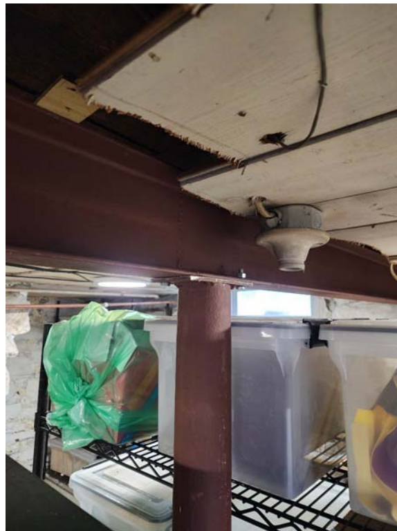
Photograph #2 (Town Hall Annex) – First Floor Shoring
