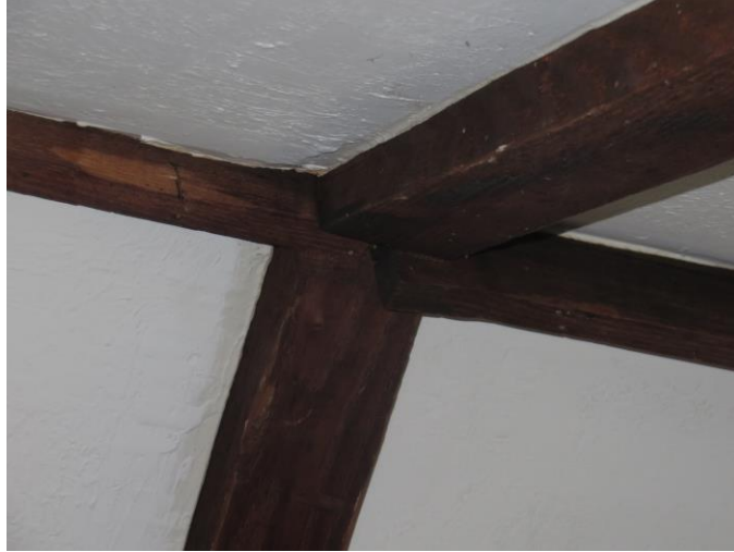
Photograph #4 – “Storage” Ridge Member
