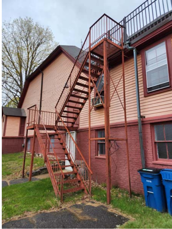
Photograph #35 (Town Hall) – Exterior Fire Escape
