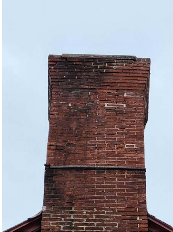
Photograph #23 (Town Hall) – Chimney Masonry
