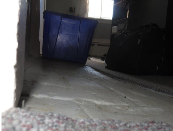
Photograph #12 – “Conservation” Sloped Floor
