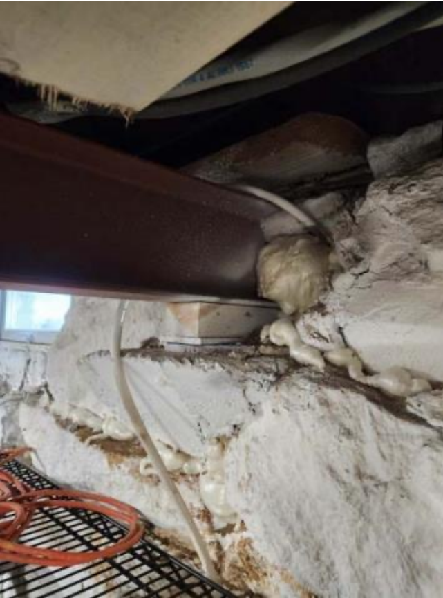
Credit: JSE 05.18.23 Structural Assessment
